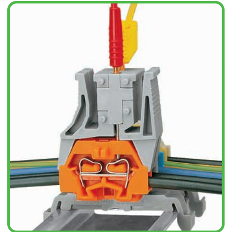
Testing terminated conductors.
